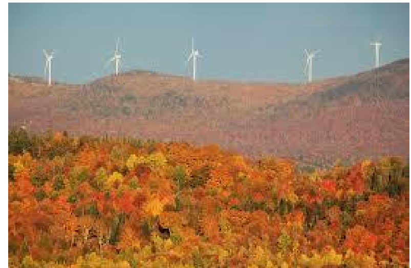
Lowell Mountain Wind Farm, Vermont
