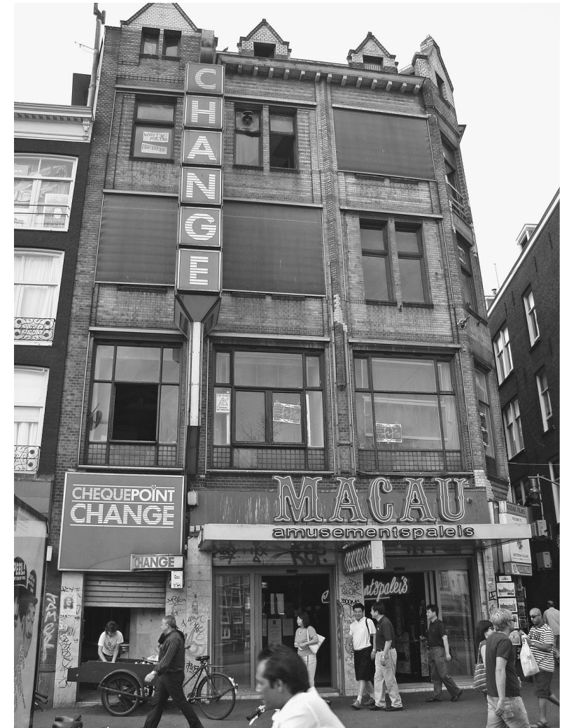
3.4 Building on the Damrak, where ground floor space was in use commercially while upper floors were squatted, 2006
