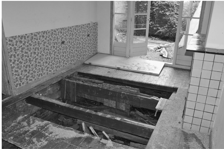
4.2 Interior of a newly squatted apartment that requires rebuilding floors, Amsterdam, 2009
