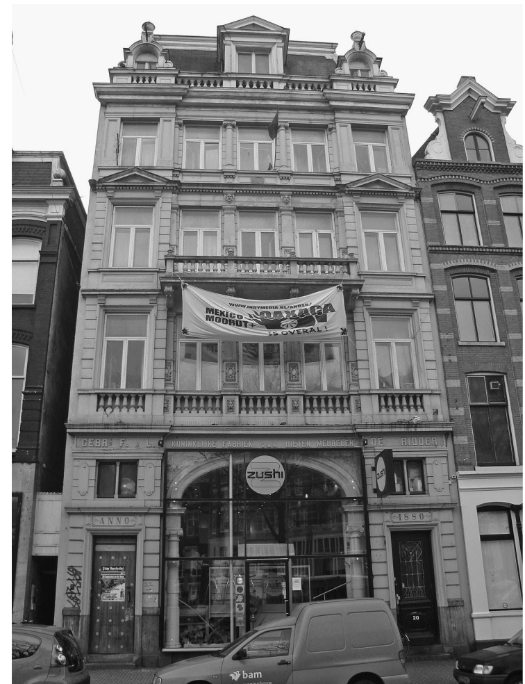
3.3 A squat alongside the Amstel River in the center of Amsterdam, 2006
