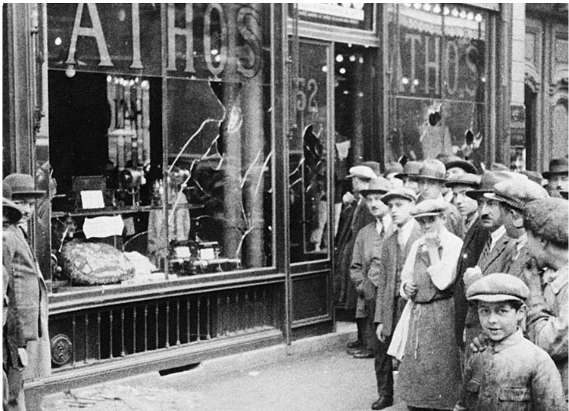
On August 23 and 24, 1927, French sympathizers smashed shop windows and wrecked places of business to vent their rage after the executions of Nicola Sacco and Bartolomeo Vanzetti. In Paris many demonstrators were injured in a clash with the police. This picture shows damage done by rioters in Cherbourg, France. Courtesy the Associated Press.
