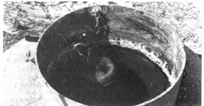
Float-valve regulates water level in stock tank.
