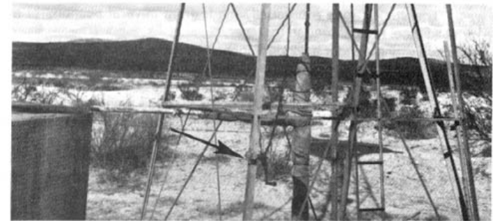
Windmill. Note windlass (arrow).
