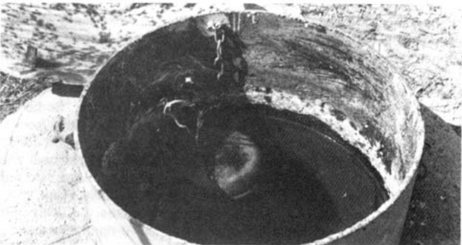
Float-valve regulates water level in stock tank.
