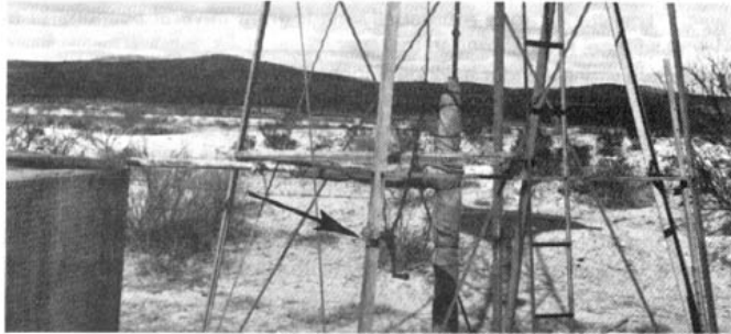
Windmill. Note windlass (arrow).
